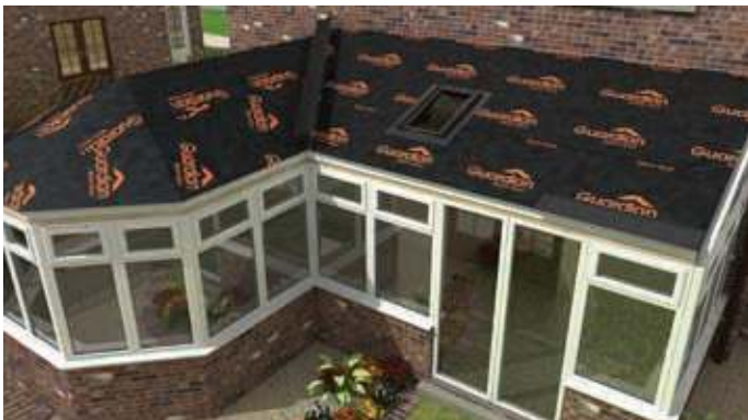
Breathable waterproof membrane is laid over the plywood and secured in place.
